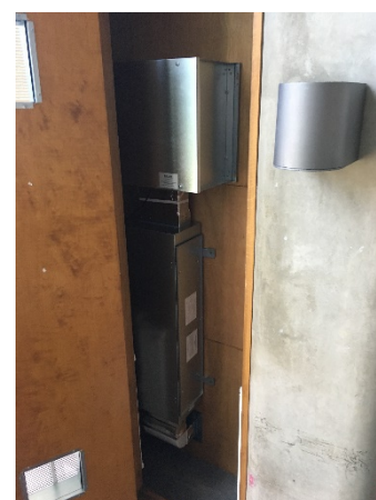
Picture 2 Air Drawn from Outside, and Filtered to Supply Fresh and Clean Air
